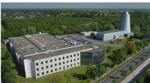
The Safran Reosc's Saint-Pierre-du-Perray space optics lab will produce the ELT M4 thin sector petals. The large astro optics plant with its 30-m tower will be equipped with new advanced large optics machinery and test means to produce the 4-m size ELT M2 and M3 mirrors.
